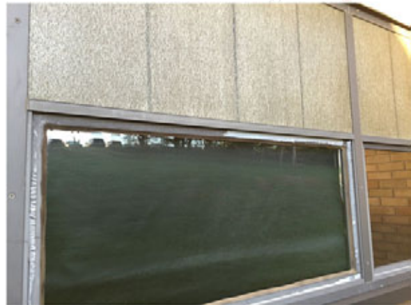
Window and Kalwall - needs replacement
