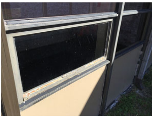
Single pane window needs to be replaced
