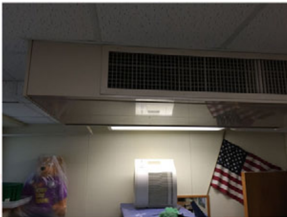
Fan coil and dehumidifier - needs HVAC update
