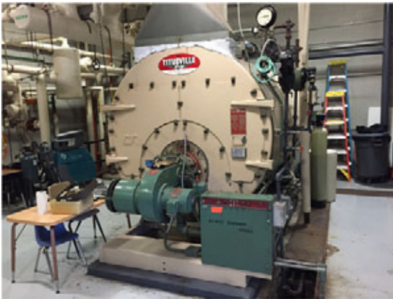
Boilers nearing end of useful life
