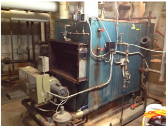
Boilers past useful life require replacement
