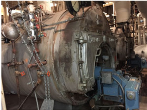
Boiler is past expected lifespan
