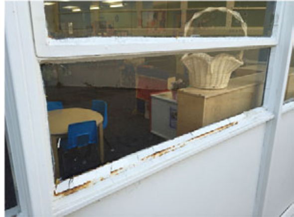
Single pane windows need to be replaced
