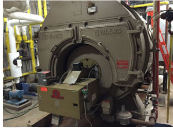
Boiler nearing end of useful life
