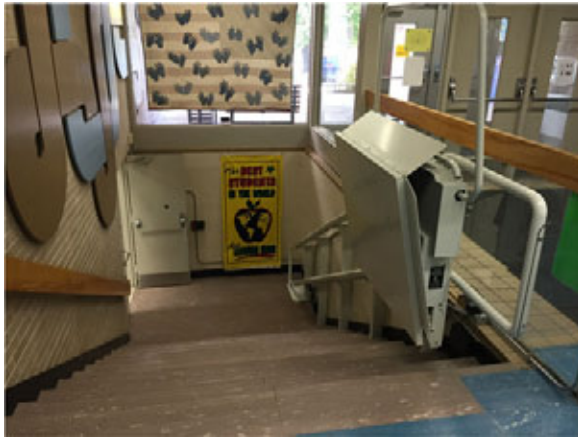
Lift from main school in narrow stair
