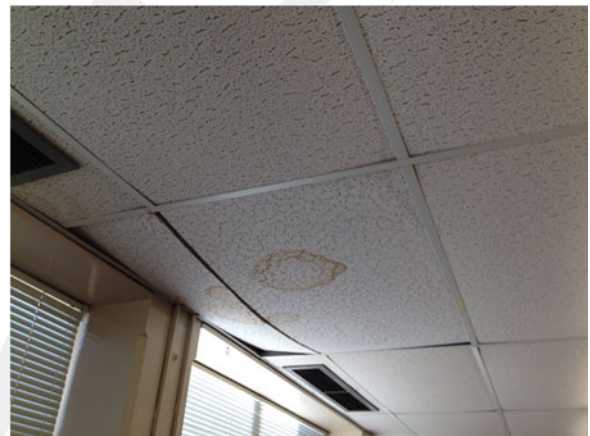
Ceiling tiles showing moisture & humidity damage
