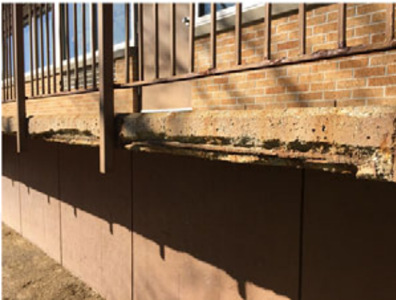
Classroom egress deck corroded
