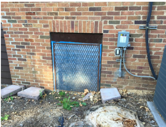
Outside air intake—requires replacement
