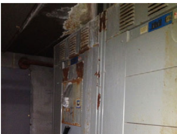
Water damage at building main electrical switch
