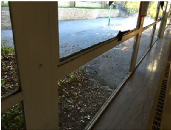
Single pane windows need to be replaced.
