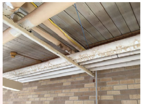
Exposed piping in hallway with condensation damage
