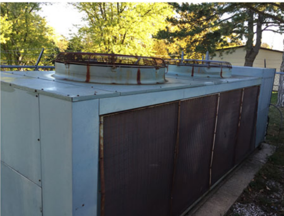
HVAC condensing unit is at end of expected life
