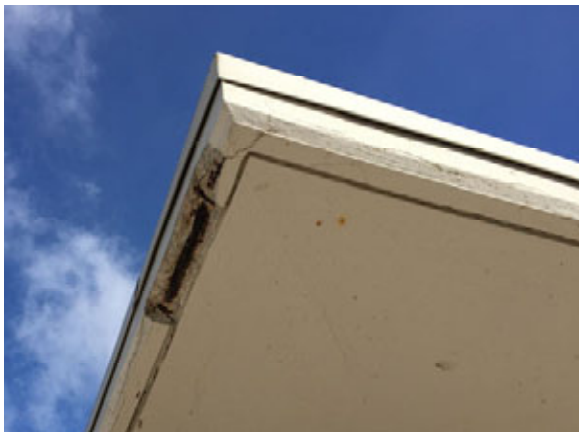
Deteriorated concrete soffit with exposed rebar
