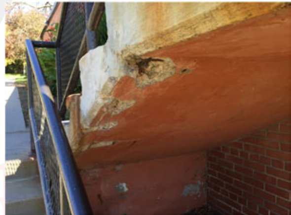
Deteriorated stair concrete needs repair
